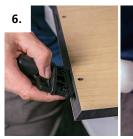
Attach the connector to the drill and alignment jig, slide it into the groove and align it with light hammer blows.
